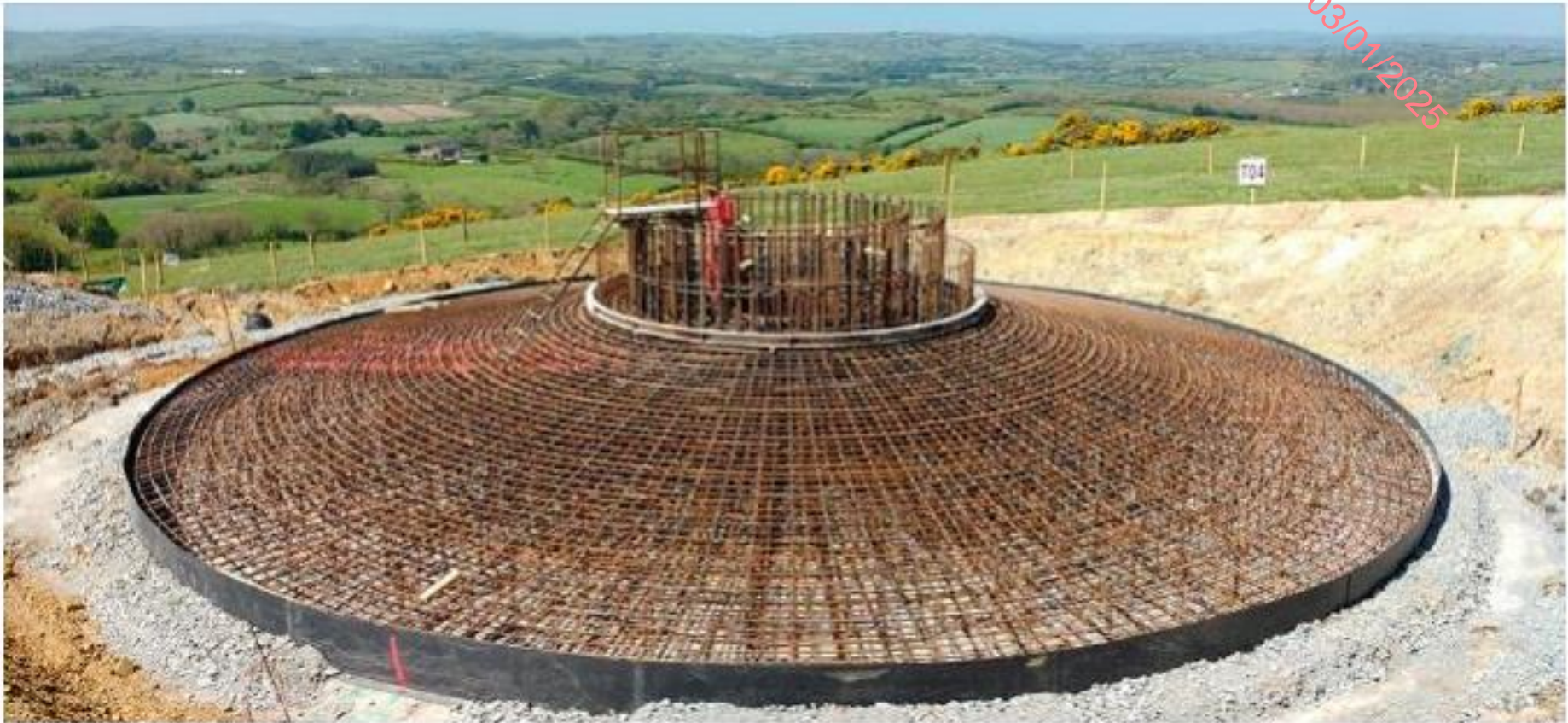
Figure 1.2 Image of a typical turbine foundation being constructed.
